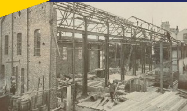
CABLE LAYING IN MARKET SQUARE IN THE EARLY 1900S
